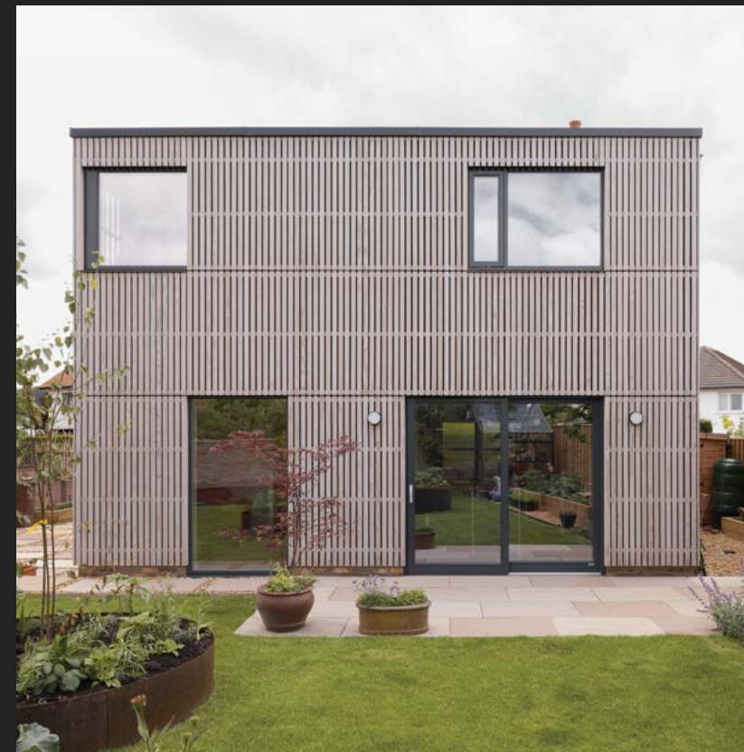
Imbue Screening, Edinburgh, Scotland. Installed 2025.
