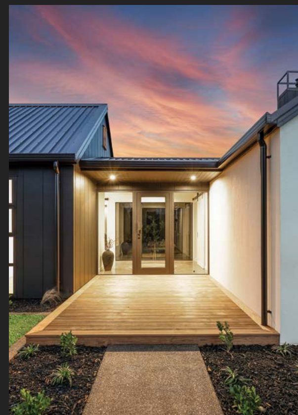
Imbue Decking, Whatawhata, New Zealand. Installed 2022.
