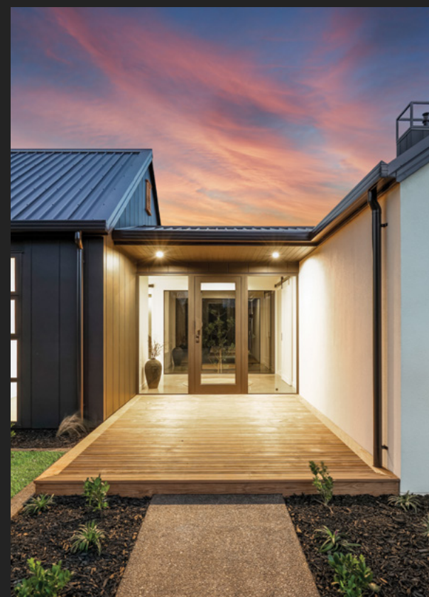
La terrasse Imbue, Whatawhata, New Zealand. Installé en 2022.
